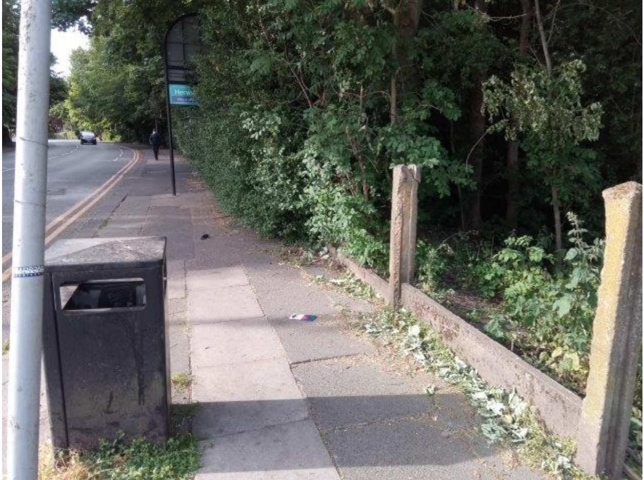
Just into Bury vegetation encroaches onto the pavement narrowing the footway.
