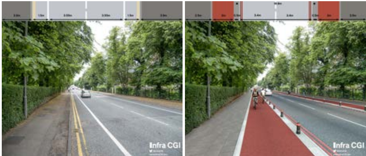
Figure 7: Bury New Road as it is (left) and as it could be with safe cycle/active travel lanes (right) courtesy of @InfraCGI on Twitter
