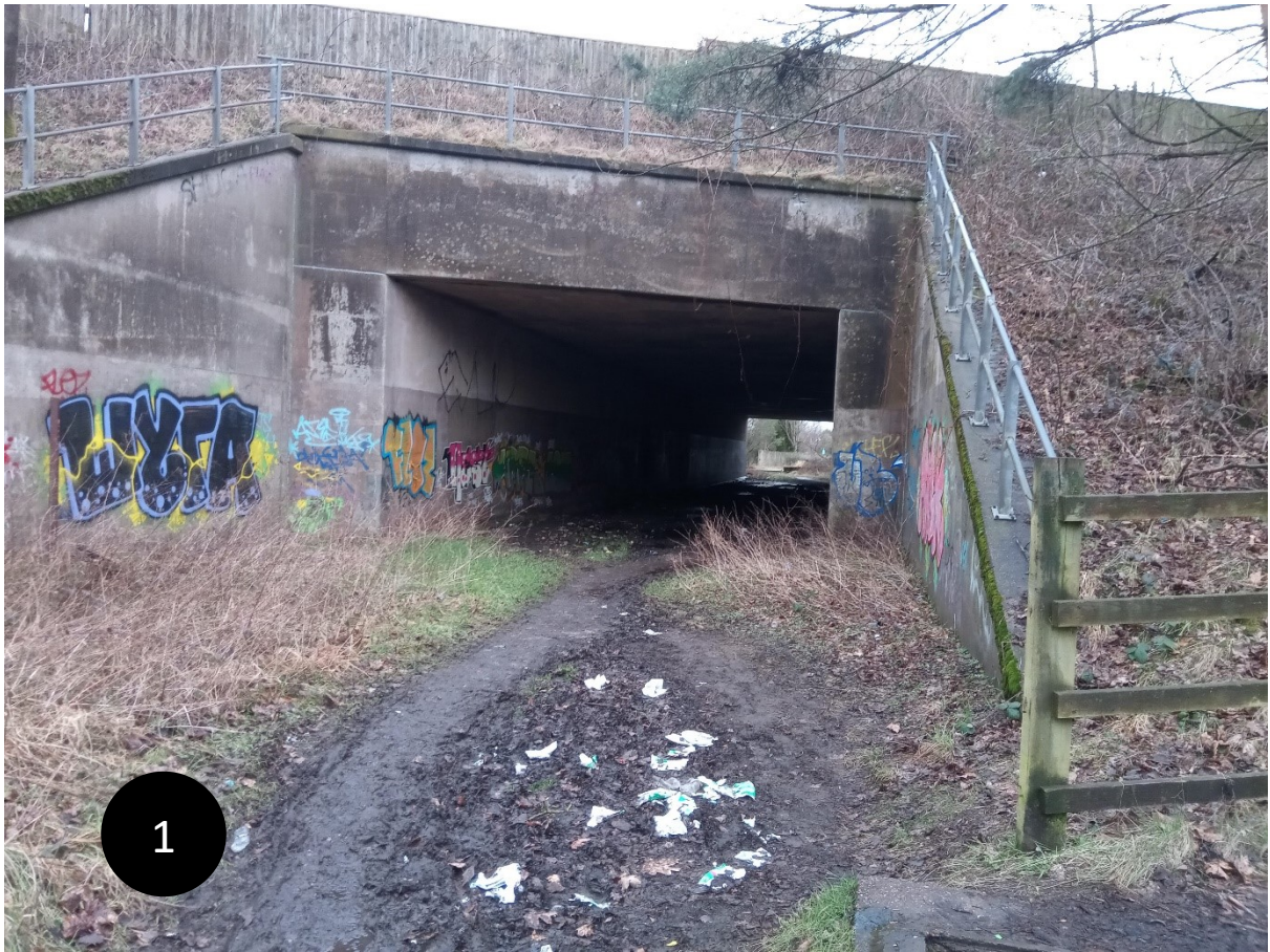
Existing M60 underpass
